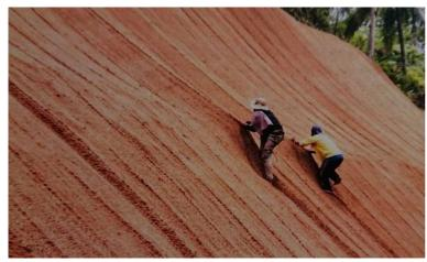
Figure 2. PIFFI members installing coconets on the scraped slopes along the newly-constructed road in Barangay Matin-ao, Burauen, Leyte
