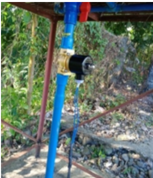
Figure 6. The solenoid valve supplying the system with water.
